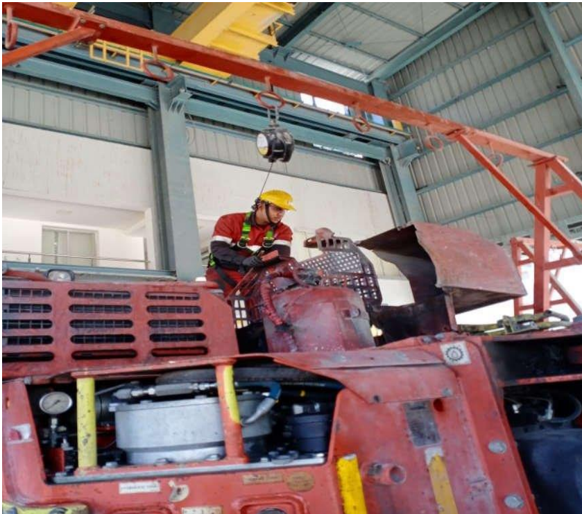
WORK AT HEIGHT USE SAFETY HARNES
